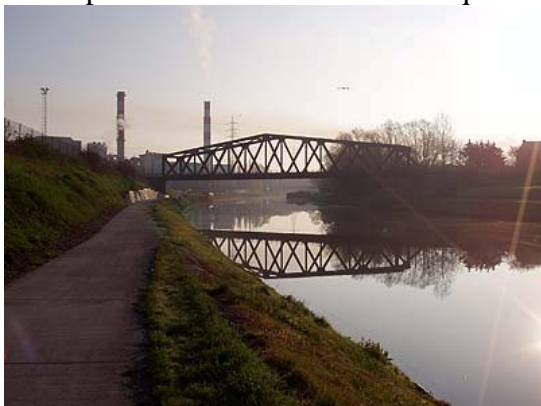
Figure 11 : Pont-rails/route de la Praye
